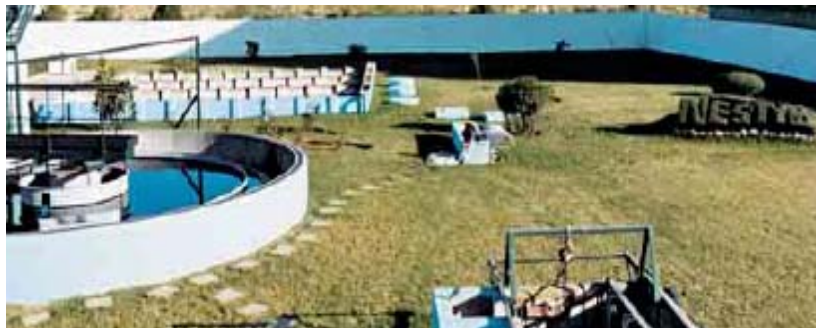
Water treatment plant, El Jadida, Morocco
