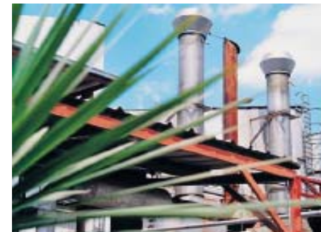
Cleaner emissions: from coal to gas, Graneros, Chile
