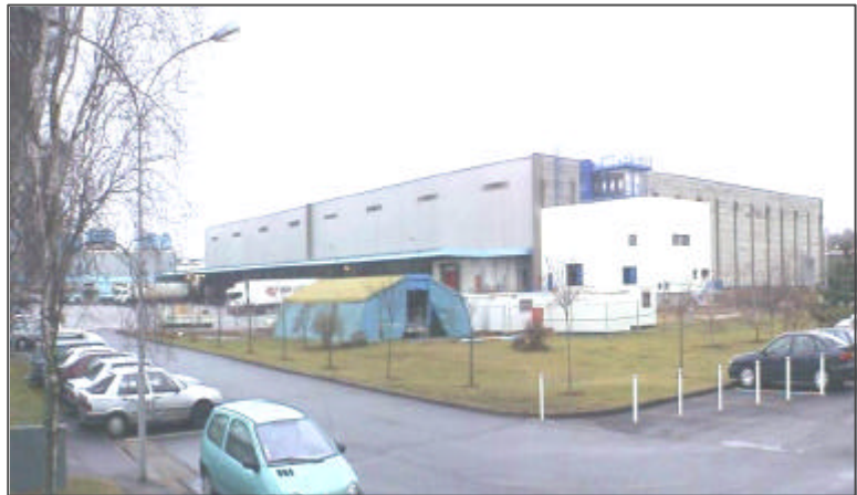
Refrigerant charge of NH 3 < 1.5 tonne / CO 2 ~6 tonne
