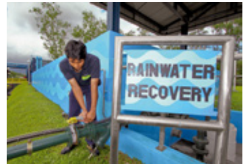
An example of environmental awareness at our Lipa factory in the Philippines, which has a system to collect rainwater from catchment areas and then reuse it in areas such as the cooling tower.
