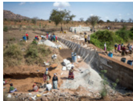
A sand dam being built by the local community.
