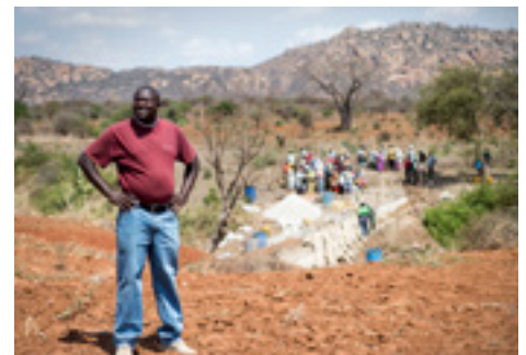
2012 CSV Prize Runner Up – Excellent Development (UK): Andrew Musila Silu, Development Director of the African Sand Dam Foundation, overseeing the construction of a sand dam.
