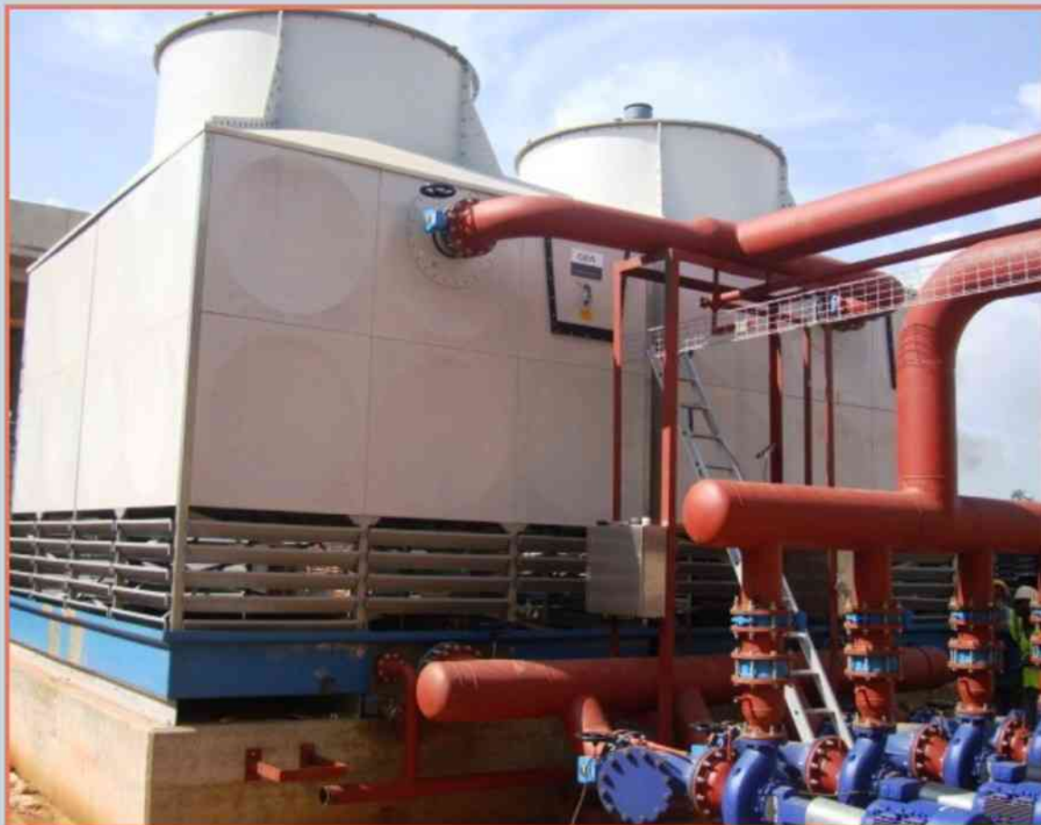
Cooling Towers at Flowergate Factory
