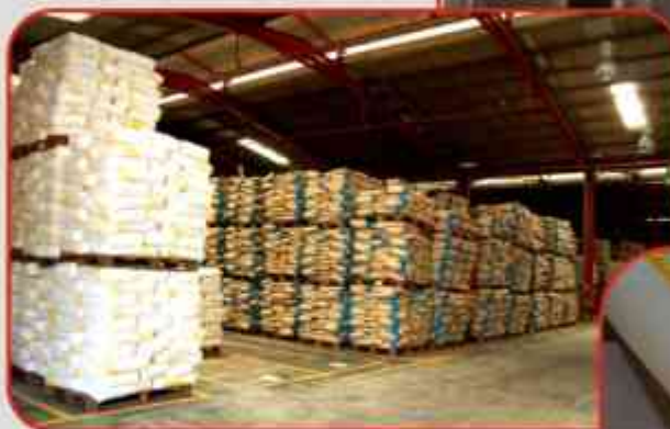
New Warehouse Extension for Raw Materials
