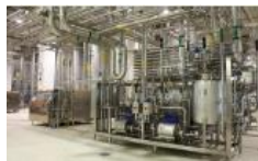
Wet blending mixing process
