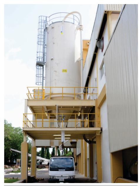
Optimising resource efficiency at Agbara factory Spent grains generated from maize, millet, soya and sorghum during processing at Agbara factory are sent to a silo, from where it is discharged to trucks, and sold to farmers for use as livestock feeds.
