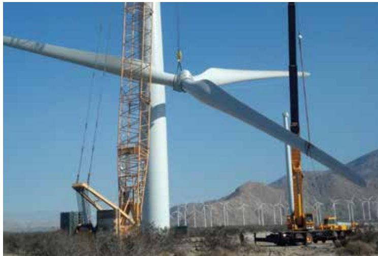
In the fourth quarter of 2012, we completed the installation of two wind turbines at our Cabazon, California plant. The turbines will generate up to 30 percent of the plant's total energy – enough to power 1,100 U.S. homes.
